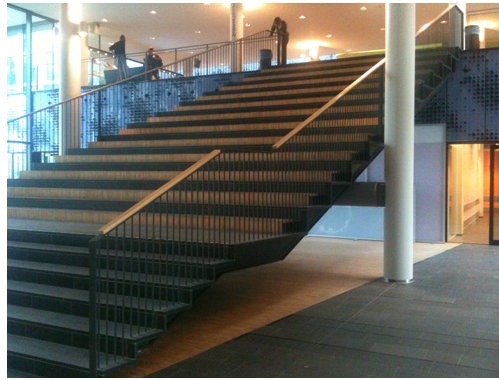
Figure 8.20: Photo of the staircase which is traversed by the AR.Drone. The depth of each step is 30\text{cm} and the height of each step is 18\text{cm} . The total height of the staircase is 480\text{cm} .
